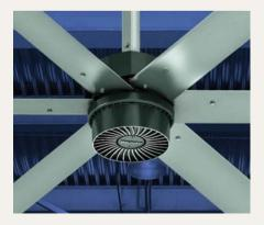
HVLS fans are generally ceiling fans although some are pole mounted. HVLS fans move slowly and distribute large amounts of air at low rotational speed.
