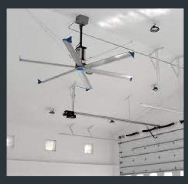
Designed with the goal of Improving air circulation, these HVLS fans replace the hot, humid air with drier air, which can prevent moisture buildup, reduce slip hazards, and allergies, and improve overall air quality. Some of the many benefits of an HVLS fan.
